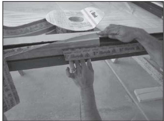
Figure 13a and 13b. Corner treatment: Illbruck Duo tape shown. Image courtesy Zola Windows.
