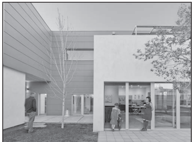
Figure 1. The south side of the residential unit. View to the living room and kitchen areas. Cement board siding and stucco. Image courtesy Mojarrab Stanford Architects (MoSA).
