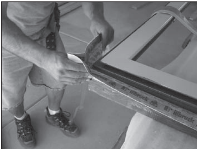
Figure 13a and 13b. Corner treatment: Illbruck Duo tape shown. Image courtesy Zola Windows.
